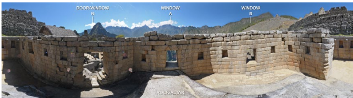
Fig. 4. Panoramic view of the upper part of the Torreón (elaborated by J. Kościuk)
