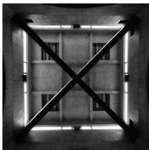
Fig. 9. The central void's roofing, 2010.
