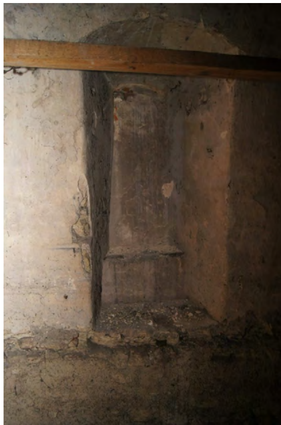
Fig. 3. Northern wall of the presbytery, view from the attic over the sacristy with the opening leading to the presbytery visible
