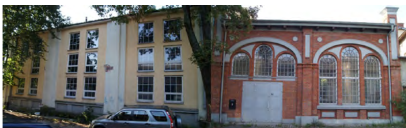
Fig. 8. Building of the boiler room and machine room – shot from 1912 repeated (Fig. 7)
