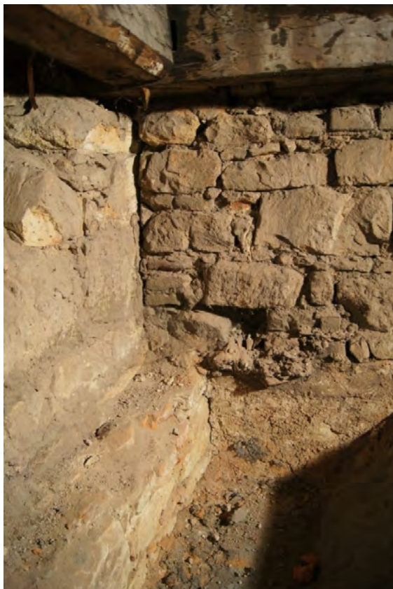
Fig. 2. View of the chancel wall from the level of the attic over the presbytery with the chancel wall visible, added to the southern wall of the presbytery
