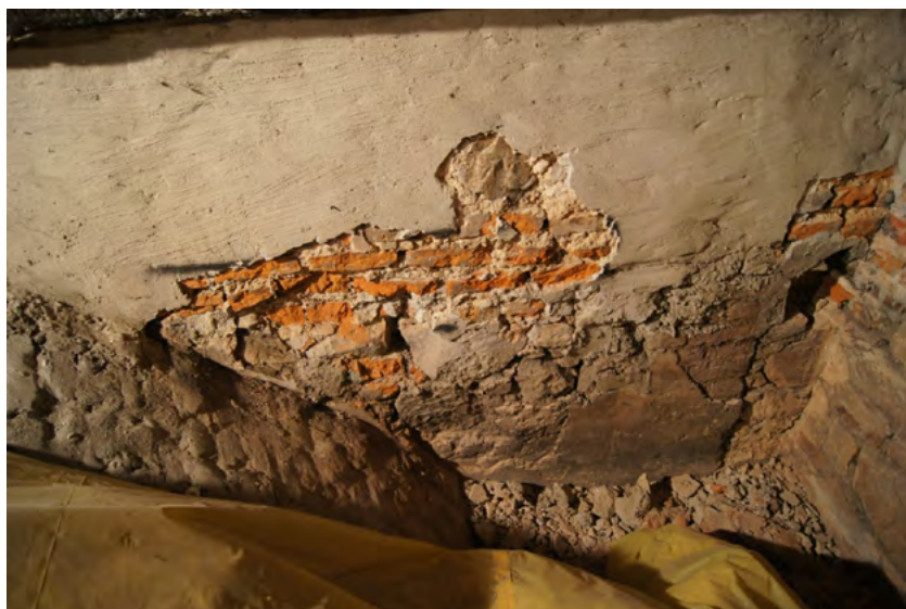
Fig. 1. View of the chancel wall from the attic over the nave with plaster relics visible, to which current vaulting was added
