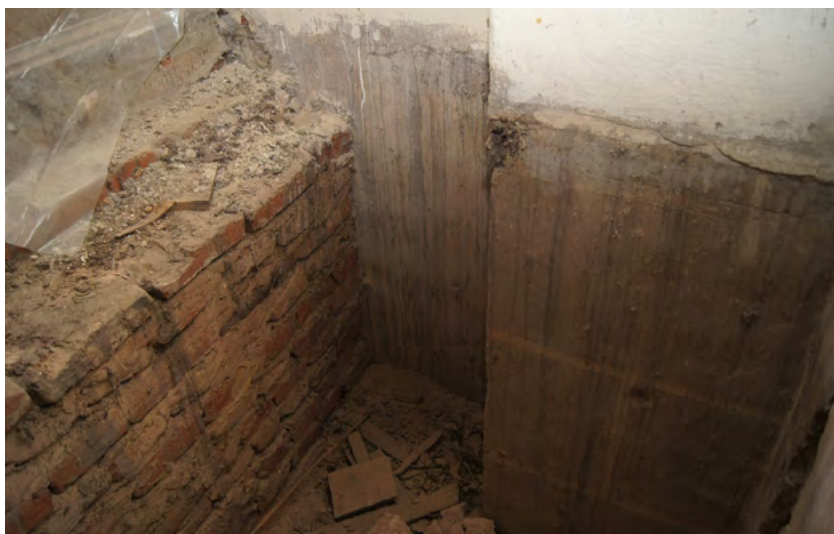
Fig. 5. Discovered paintings of nave walls and pilasters after removing the floor of choir loft arcade
