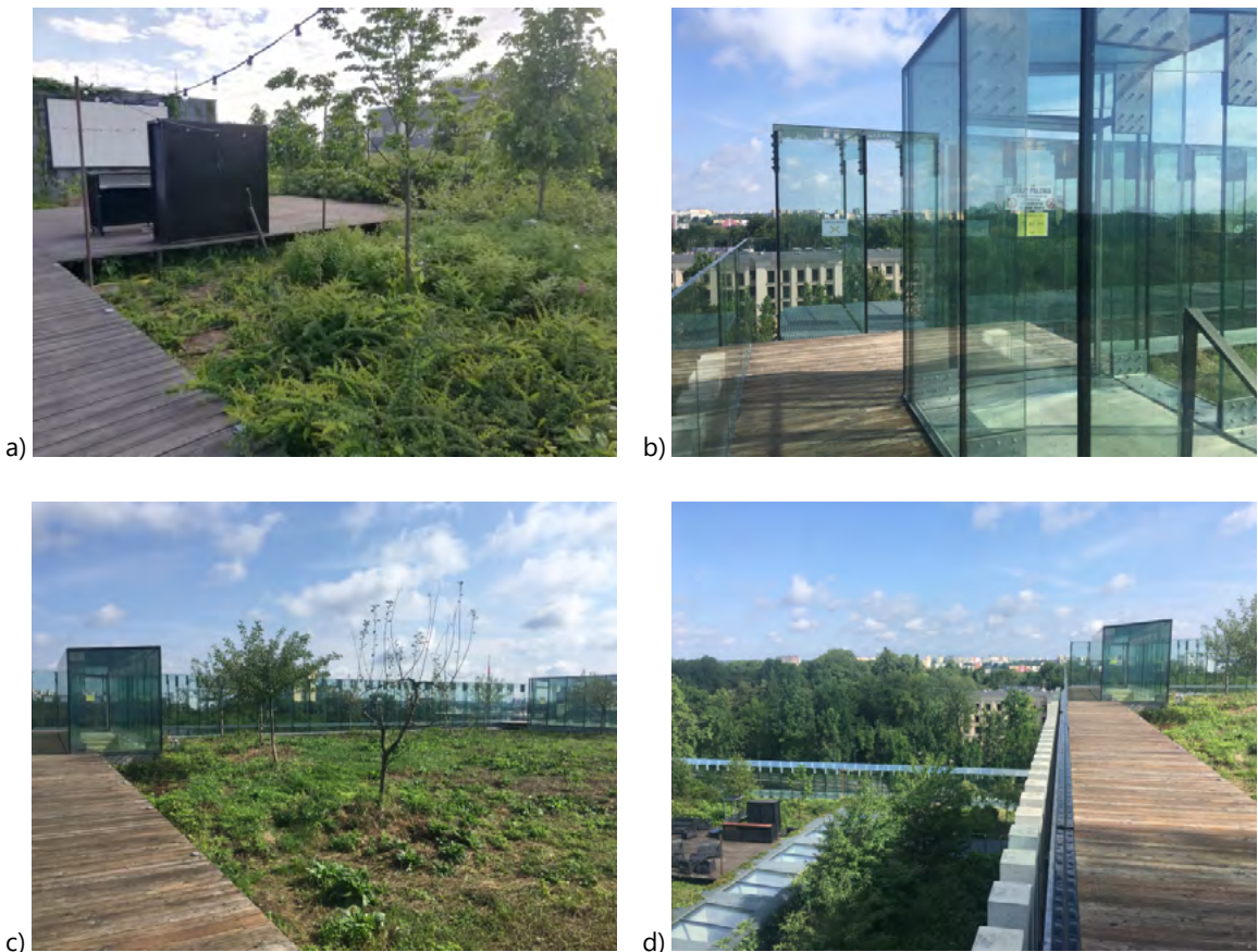
Fig. 5. Characteristic elements of the roof of the Meeting of Cultures Centre “Sky Terraces” (a) – arrangement for temporary attraction, (b) – entrances and glass tunnels, (c) – main walking path, (d) – general view
