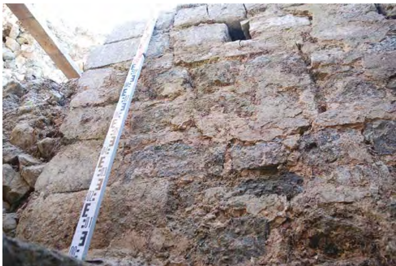
Fig. 6. The outer face of the western wall of the palatium – demonstrates the method of laying hewn blocks in the wall; excavation 35 (photo by S. Gołub)
