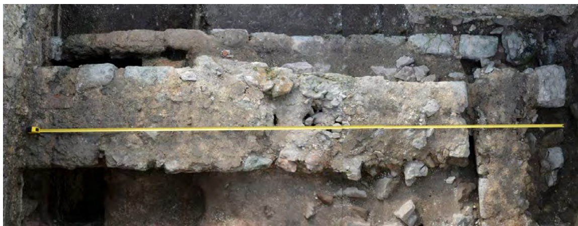
Fig. 3. A wall of glauconite blocks in the archeological excavation of building D in the northern part of the castle. Photo by S. Gołub
