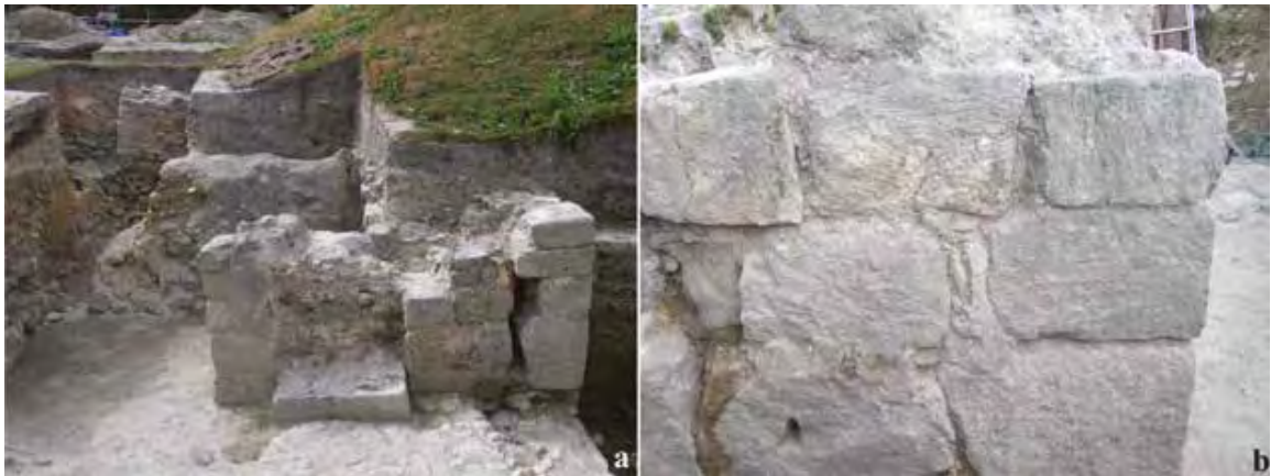
Fig. 2. Preserved elements of buildings made of glauconite: a – the entrance gate to the palace part of the castle, b – a fragment of the wall around the perimeter of the southern part, built of glauconite (photo S. Gołub)
