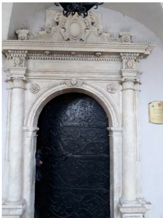
Fig. 3. Portal in the The Birkowski tenement house, Rynek Wielki 6, author's photograph
