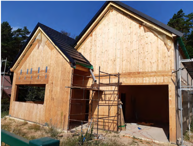
Fig. 2. Building in a wooden structure. Own photo
