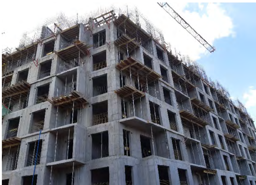
Fig. 1. Reinforced concrete structure. Own photo
