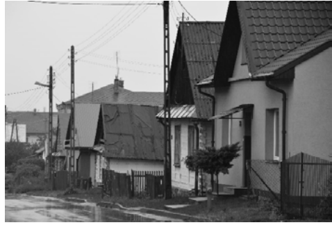
Fig. 3. Remains of Frampol's wooden buildings. (photo by Sosnowska)
