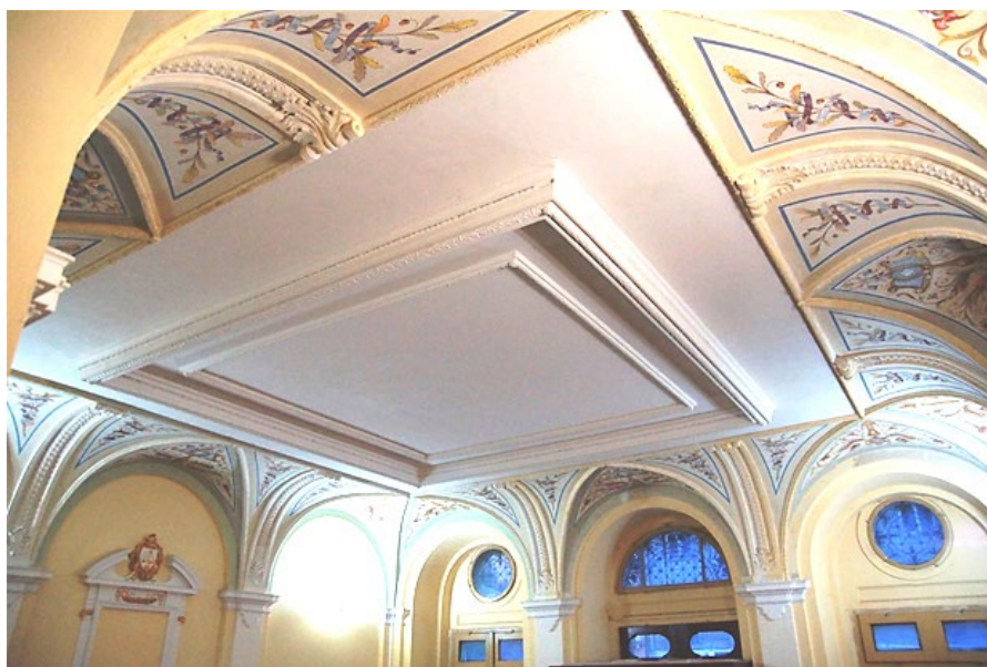
Fig. 17. The main lobby of the 19 th academic building of L'viv Polytechnic National University in 2015 after the completion of reconstruction and restoration works (photo by M. Bevz).
