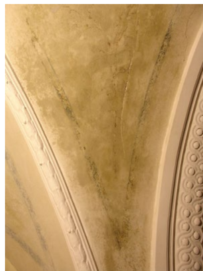
Fig. 4. Saved under a later covering a fragment of art paintings of the XIX century (photo by M. Bevz).
