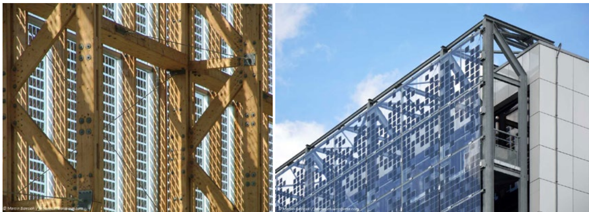
Fig. 8. Binary modules visible from inside Mont-Cenis Academy, Herne (arch. Jourda et Perraudin, 1999), and from outside in GDF Suez, Dijon (arch. Atelier Phileas, 2013) – photographs by M. Muszyńska-Łanowy.
