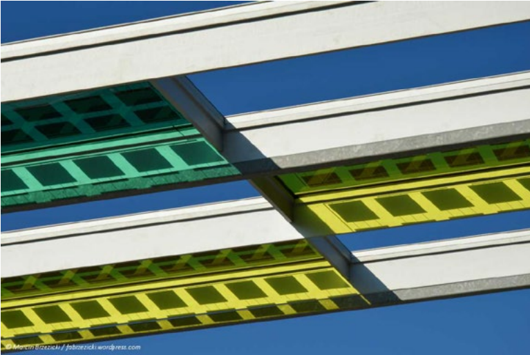
Fig. 5. The glass PV module with color PVB resin shading element at Parc de Can Rigoal, Barcelona (arch. Claudi Aguiló Riu, Eva Pagès (arquitectos – AMB, 2012) – photographs by M. Muszyńska-Łanowy.
