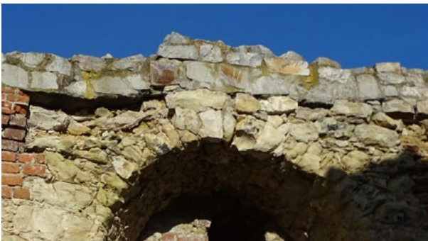
Fig. 2. Photo 1 Bricklaying the crown of the wall with a quartzite stone
