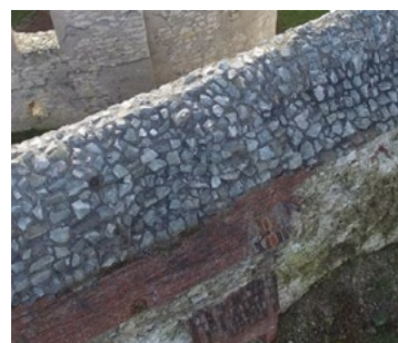
Fig. 5. Photo 3 Shaping the crown of the wall
