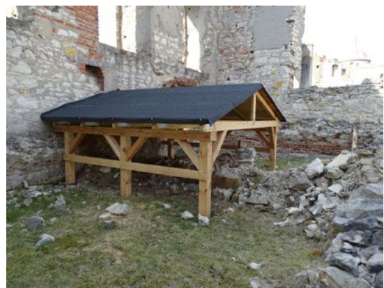
Fig. 9. Photo 6 Shaping the crown of the wall
