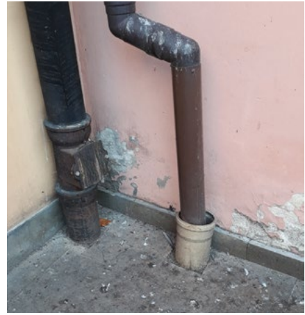
Fig. 9. Courtyard No. VI Down pipes 'sinking' beneath the ground connected to sewerage closed system; Source: author's own photo
