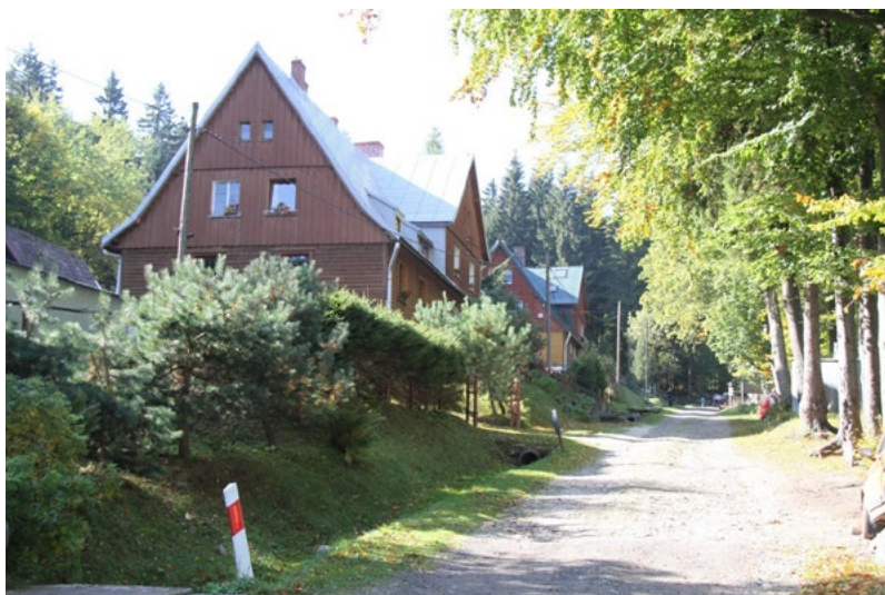
Fig. 12. Zieleniec. Leśne Apartamenty , former border guard buildings from the 1930s, now adapted to the leisure function. Photo by the author – 2017.
