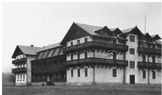
Fig. 3. Tatarów, Policemen's Health Center, ca. 1930 Archival photo [AAD-ZZS, sign. 112].
