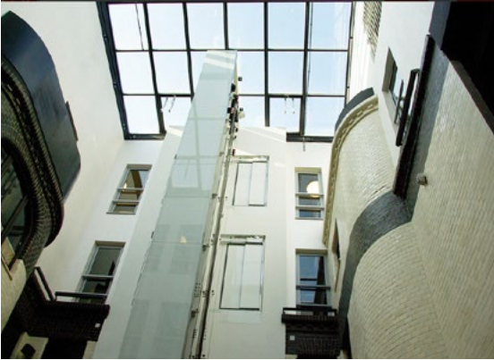
Fig. 20. The multi-story atrium of Hieronimus I Office Building refurbished in accordance with the design by Grupa 33_03 – a view showing the new glazed elevator shaft (photo by Grupa 33_03).
