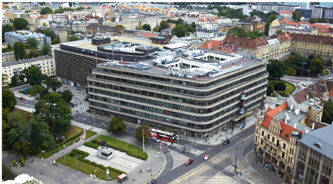
Fig. 17. The Renoma Department Store refurbished and extended in 2005–2009 – top view, ventilation ducts visible on the roof of the building (photo by Fotopolska).
