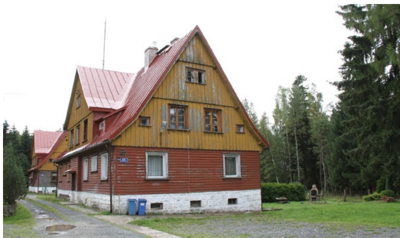
Fig. 18. Border guard buildings erected in 1938 in Lasówka. The proportions of the whole and architectural detail indicate the regional character of the objects. Photo by the author. 2017.
