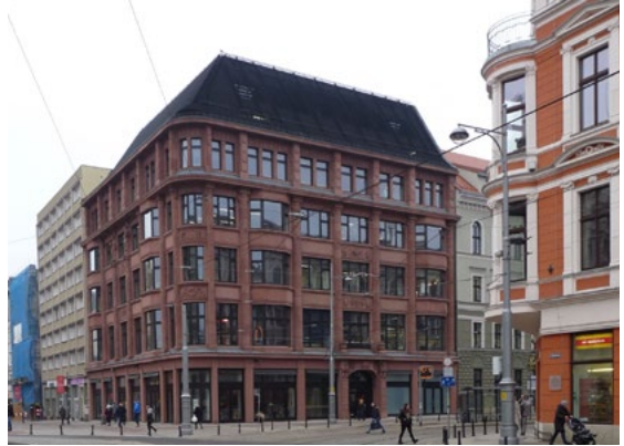
Fig. 21. Hieronimus I Office Building refurbished in 2015 in accordance with the design by Grupa 33_03 – view from the South (photo by P. Kirschke).
