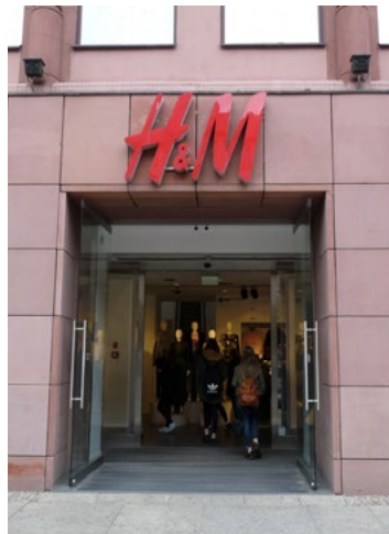
Fig. 7. The main entrance to Hennes & Mauritz department store (H&M) refurbished in 1997–2004 in accordance with Studio EL design (photo by P. Kirschke).
