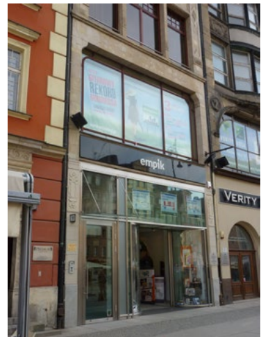
Fig. 8. The main entrance to EMPiK building refurbished in 2012 in accordance with Kirschke Pracownia Projektowa (photo by P. Kirschke).
