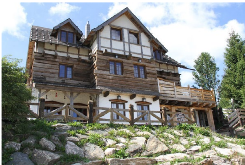
Fig. 10. A recently constructed guesthouse in Zieleniec with quite surprising structural and formal solutions of external walls. The transom system of attic beams contrasts with the wooden and log load-bearing system of the first floor (recycled building material), and brick walls (?) of the ground floor. Photo by the author – 2017.
