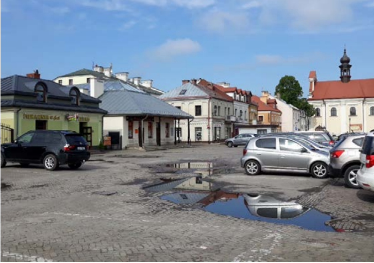
Fig. 12. Uneven clinker surface in the parking area, 2–3-step difference in the areas of the entrances to the groundfloor shops and services, Zamość, The Stefanidesa Square. Photo: Katarzyna Kielin
