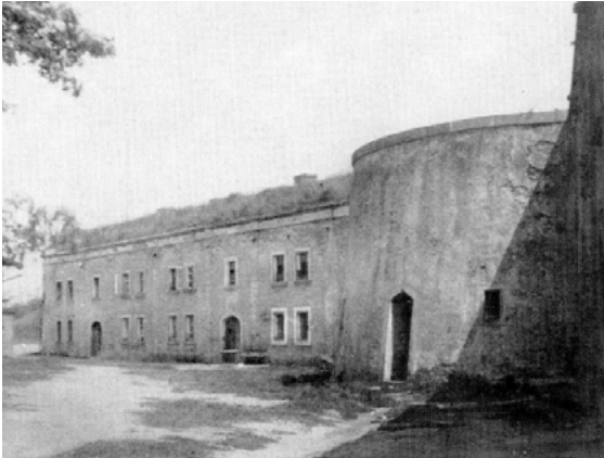
Fig. 3. The front elevation of the northern part of the former Red Barracks (1910–1920) (source: https://polska-org.pl ).
