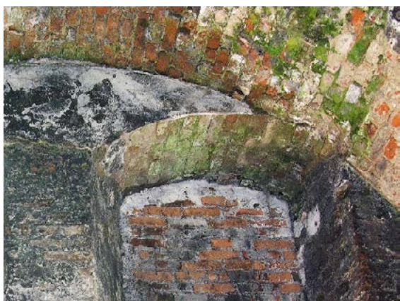
Fig. 23. Room No. 27. Mosses, lichens and salt efflorescence on the window lintel and vault.
