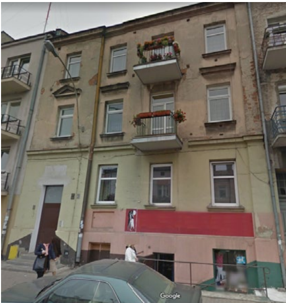
Fig. 10. Tenement house 4, www.google.com/maps/ street View , state of 2011, access: 15.08.2019
