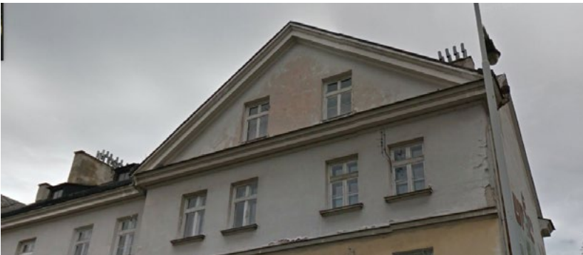
Fig. 14. Tenement house 4, www.google.com/maps/ street View , state of 2011, access: 15.08.2019
