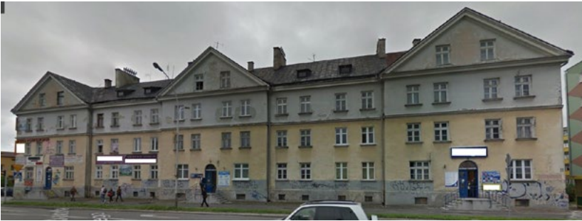
Fig. 12. Tenement house 6, www.google.com/maps/ street View , state of 2011, access: 15.08.2019
