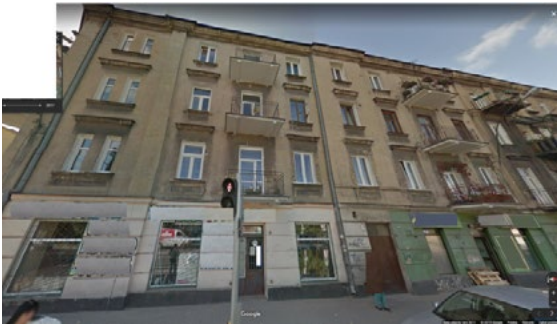
Fig. 6. Tenement house 3, www.google.com/maps/ street View , state of 2011, access: 15.08.2019
