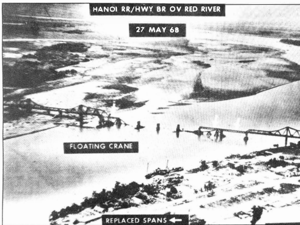
Most Doumiera w Hanoi po jednym z ataków ● Doumier's Bridge in Hanoi, after one of the attacks
